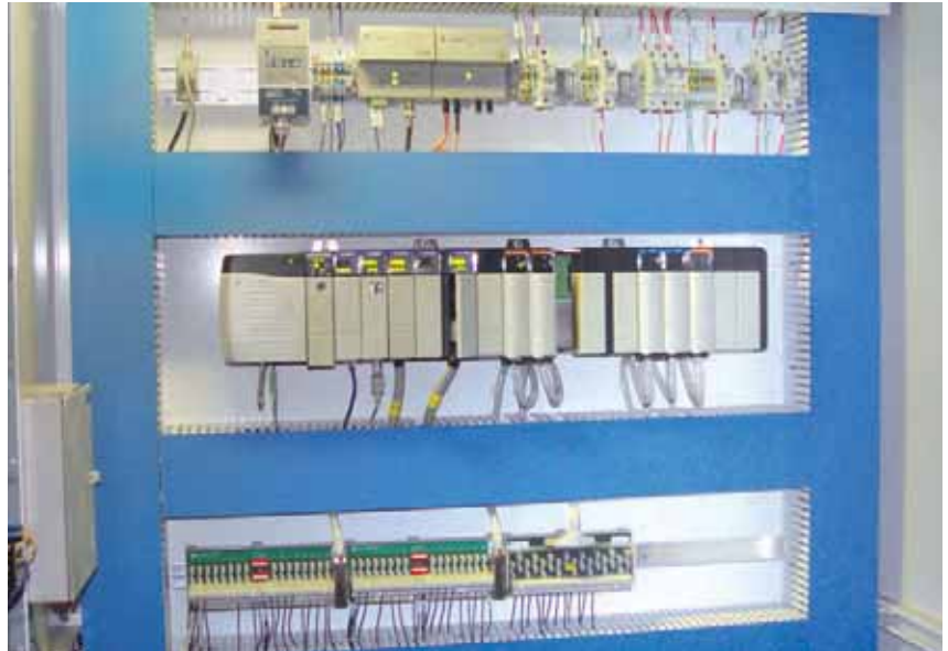
This control panel at U.S. Sugar includes an Allen-Bradley ControlLogix PAC, DeviceNet cards and other I/O cards.
